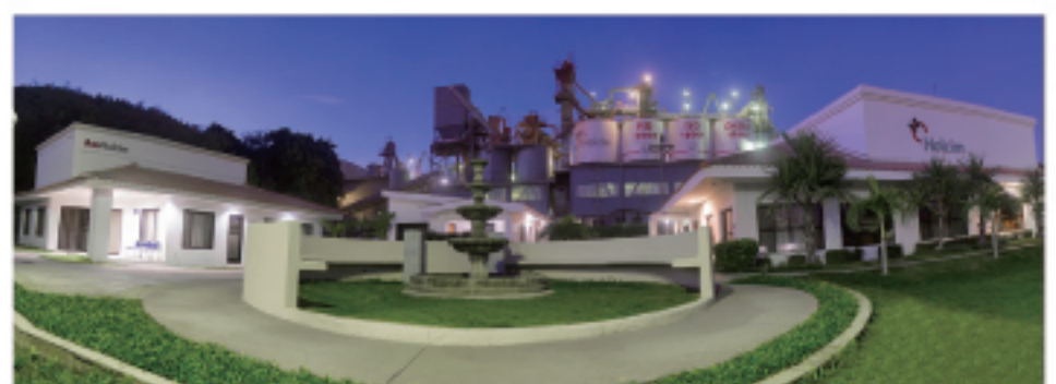
Nagarote, Cement Plant.
