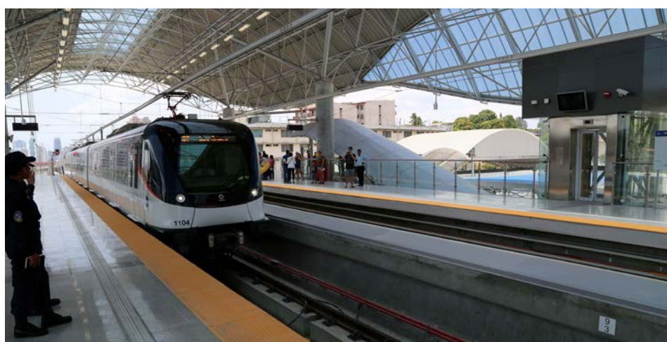
Panama Metro, Line 1.
