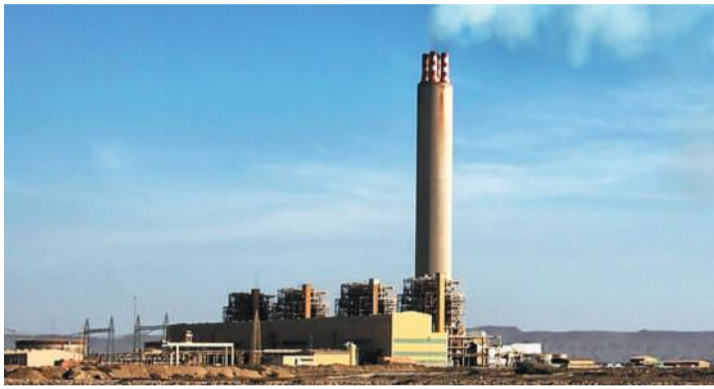
One of Hub Power Companies thermal power plants providing 1200 MW of reliable power to the national grid of Pakistan.
