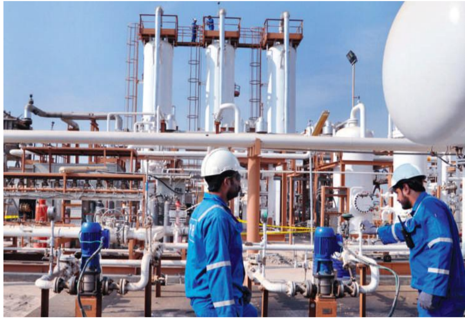
Gas Processing Facility IV, Gambat South.
