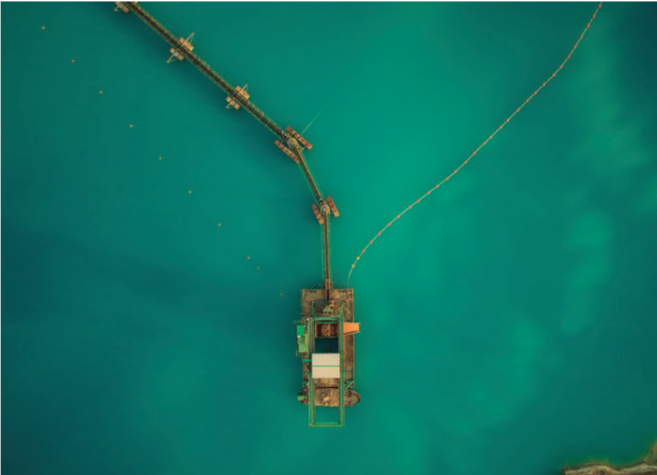
Dredging & Land Reclamation.
