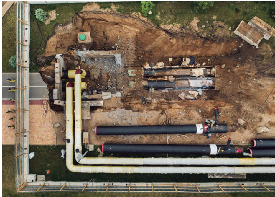
Pipeline Installation & Maintenance.
